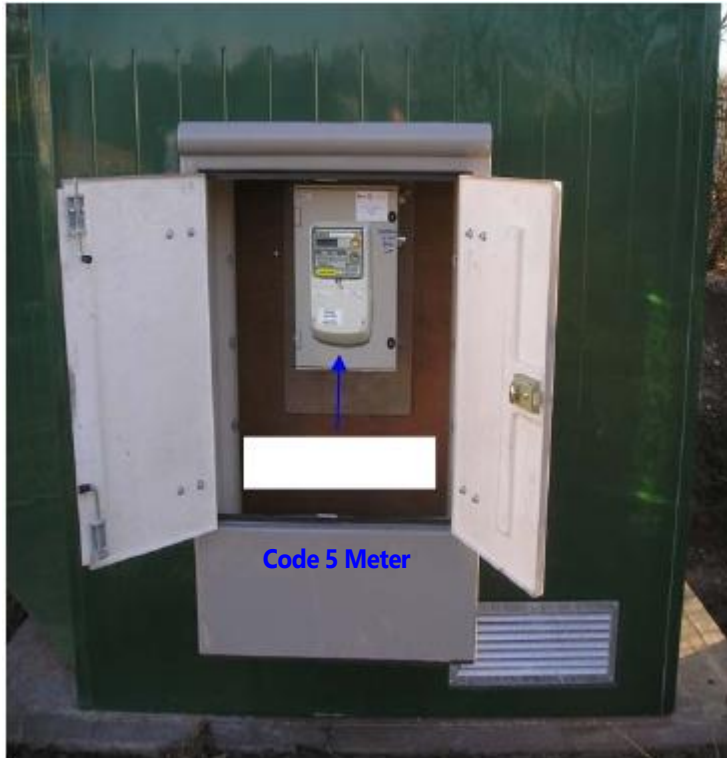
Internal view of GRP Housing attached Code 5 or Code 3 Metering Cubicle showing Code 5 Meter
