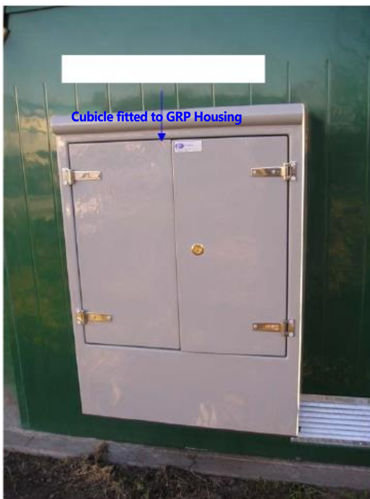
External view of GRP Housing attached Code 5 or Code 3 Metering Cubicle
